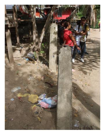
Figure 4. Washed Out Column
